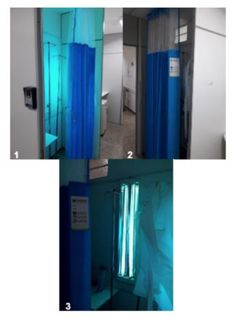
**Figure 2.** ""UVC closet" with motion detector device at different agles (1, 2 and 3), for disinfection of gowns in the COVID-19 area: two UVC lamps of 60W each.
